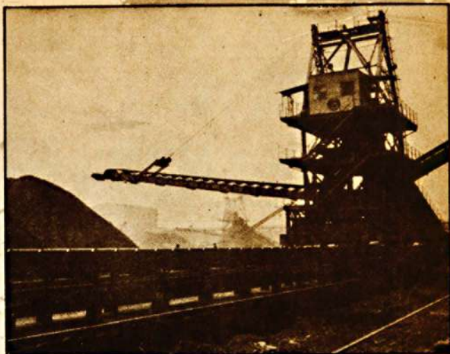
Bokaro's raw-material handling yard: this gigantic 'stacker' piles raw materials in heaps, as on the left, after they have been sorted and blended alongside; this method of raw-material processing, which exists elsewhere only in Durgapur, vastly improves steel plant operations.
