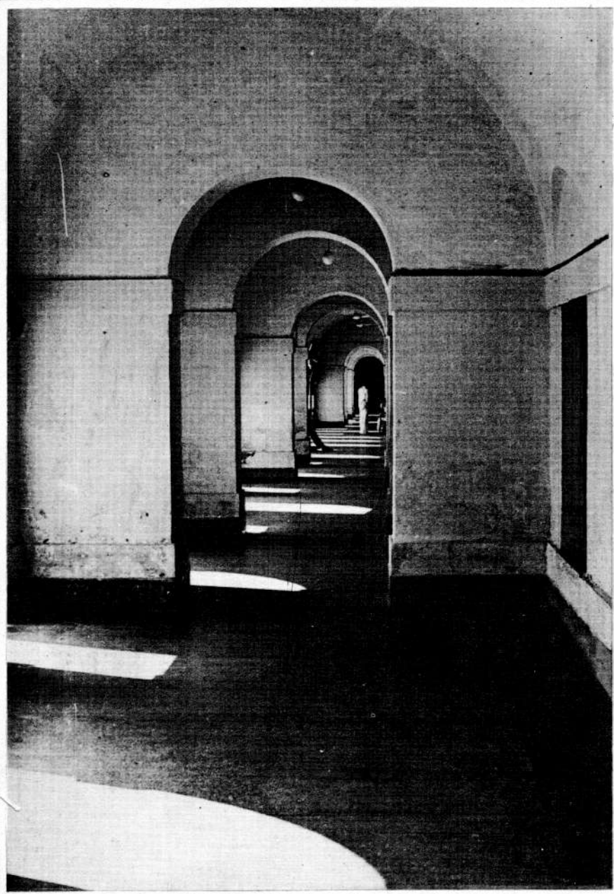
Sunlight shows up rising damp in decaying colonial arches
