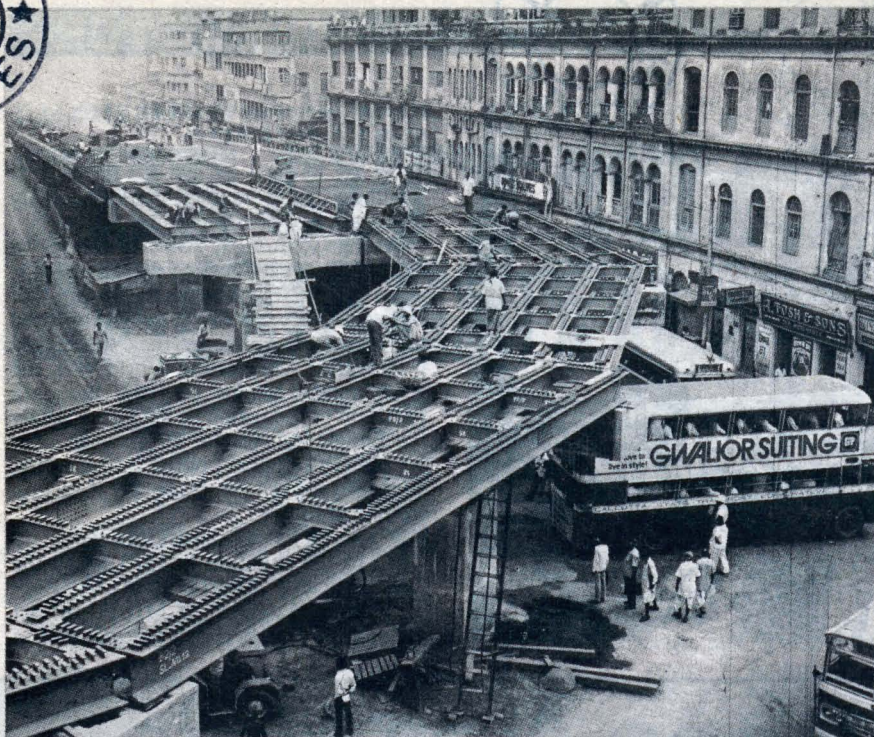
FLYOVER BEING CONSTRUCTED AT BRABOURNE ROAD TO RELIEVE LOAD ON APPROACH TO HOWRAH BRIDGE
